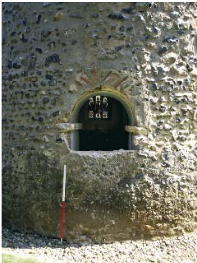
Plate 6 Howe: The partially unblocked western door of the church.
