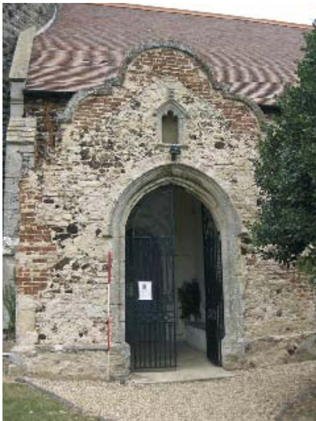
Plate 12 West Dereham: The porch of St Andrew's church.
